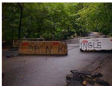
Barricaded Klingle Road, on the Porter Street side.
